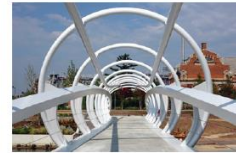
NEW PEDESTRIAN BRIDGE
