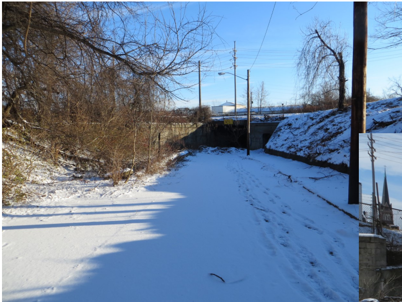
Booth Ave. Underpass
