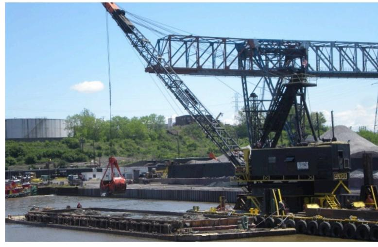
FIGURE 20. A CRANE WITH A CLAMSHELL DREDGE PLACING MATERIAL IN A DREDGE SCOW.
