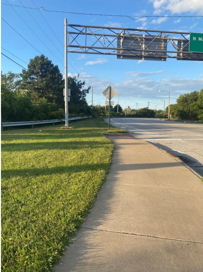
Sidewalk ends, forcing crossing in high speed road segment
