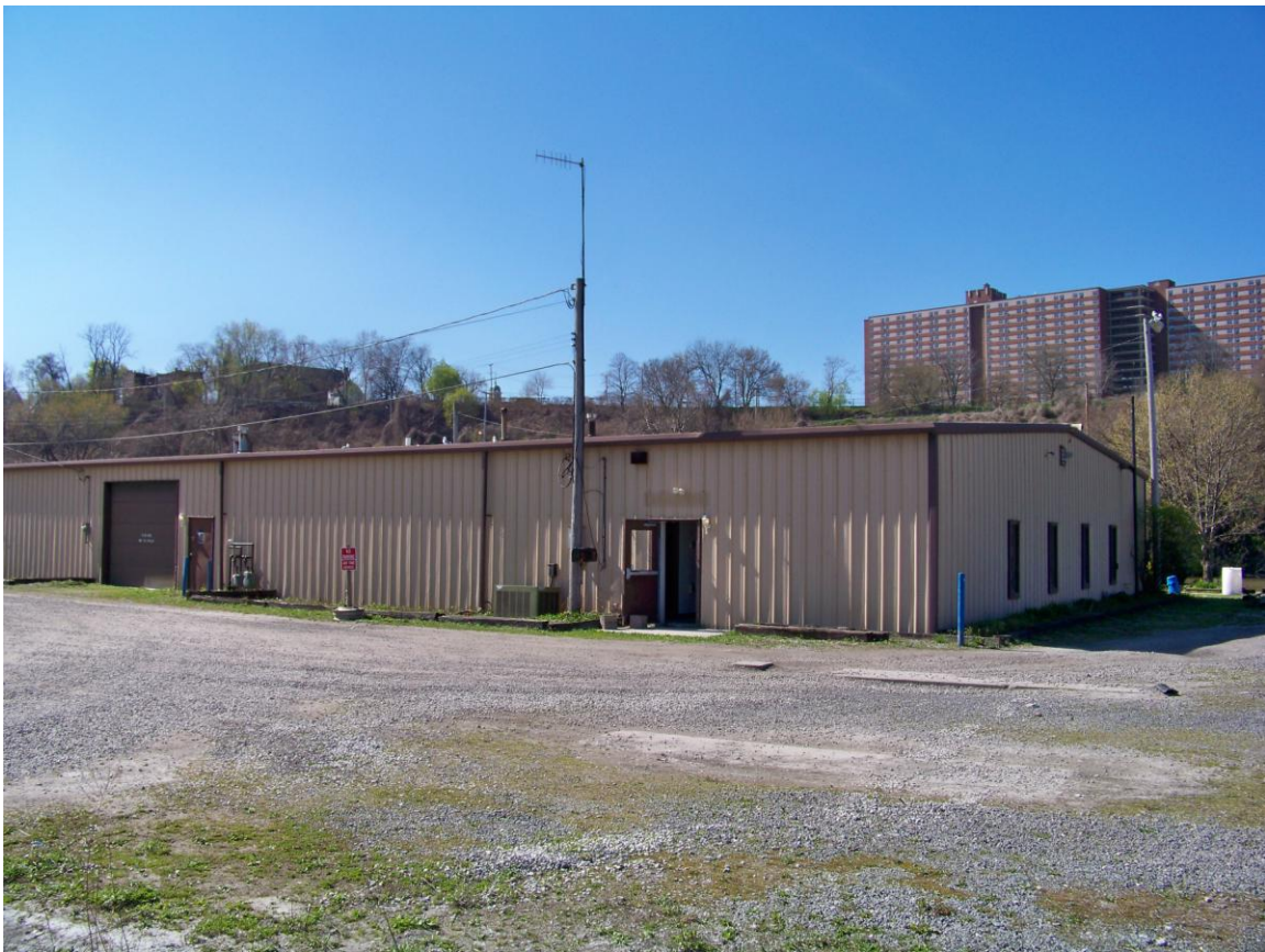
Rivergate Building – Exterior Views
