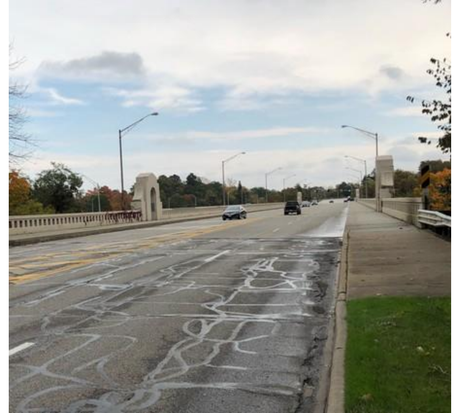
Hilliard Road bridge deck
