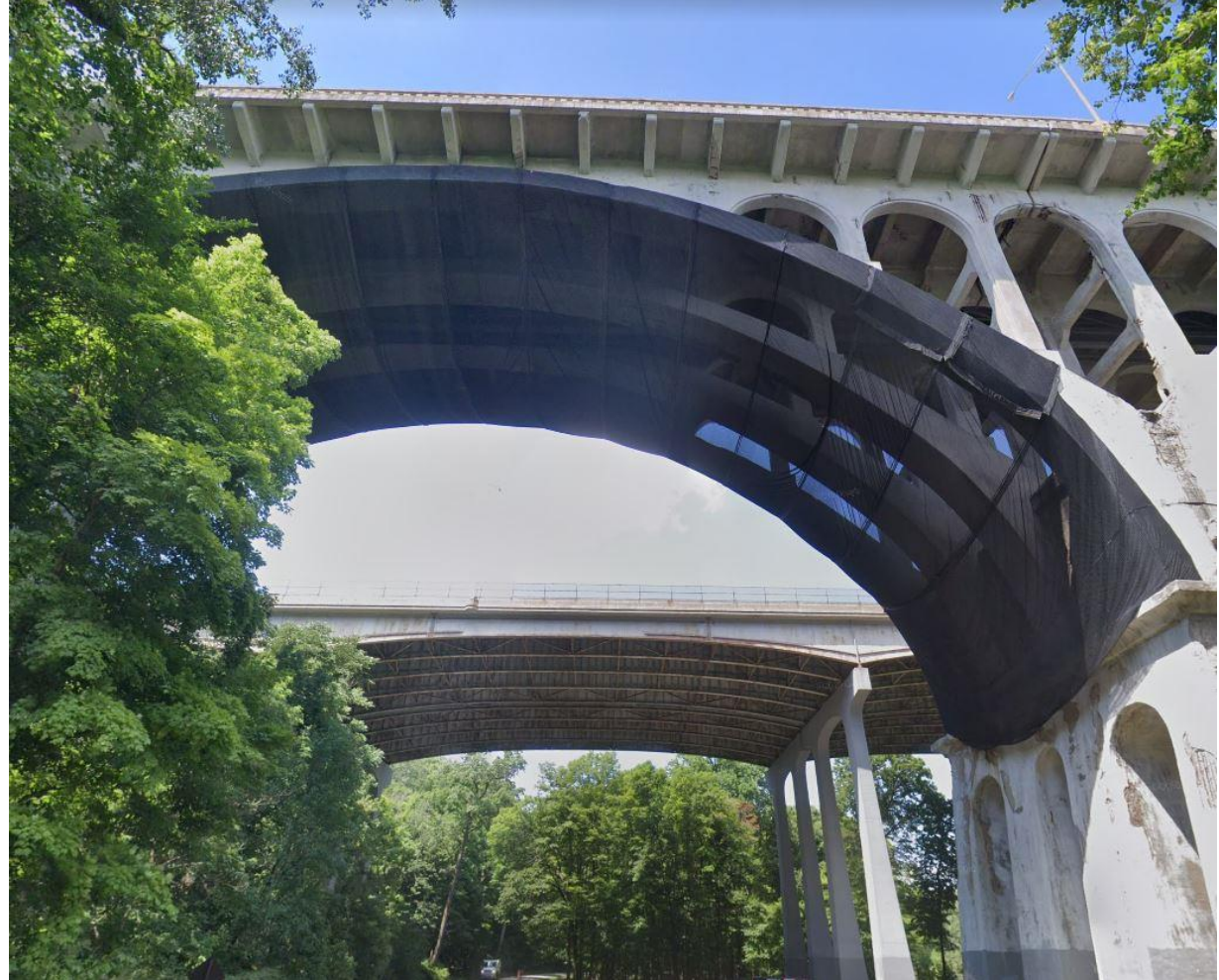
Safety netting installed to protect traveling public from falling concrete debris
