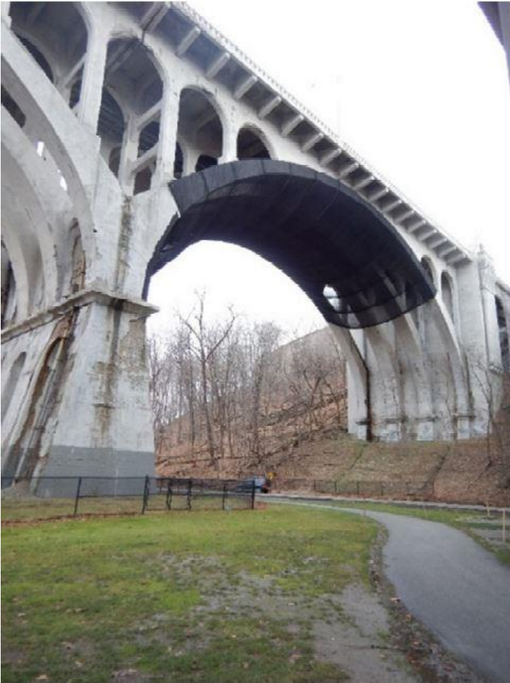
Safety netting installed to protect traveling public from falling concrete debris
