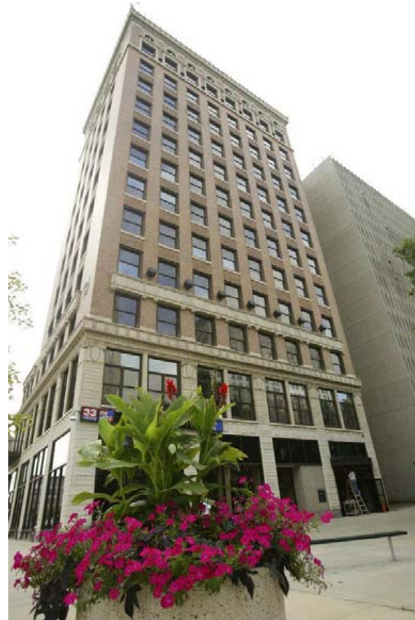
Realty Building and Wick Building City Architecture
