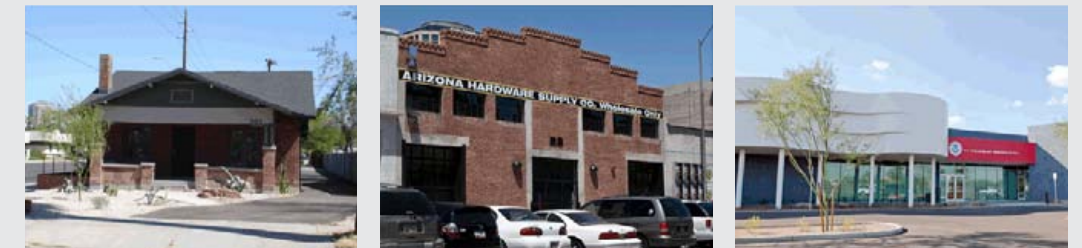
Phoenix, Arizona: Images of buildings rehabilitated under Adaptive Reuse program City of Phoenix, Office of Customer Advocacy (Adaptive Reuse Program), http://www.phoenix.gov/pdd/services/permitservices/arp.html
