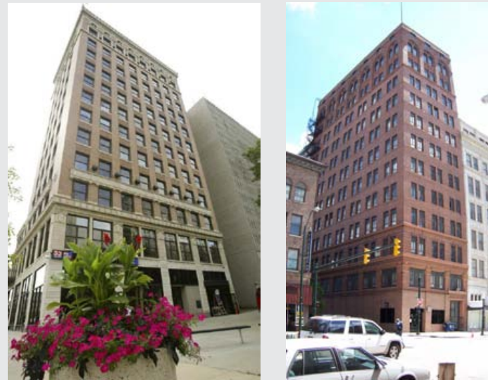
Realty Building and Wick Building City Architecture
