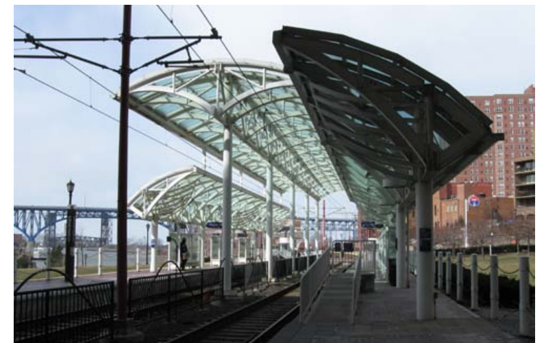
GCRTA Flats East Bank Rapid Station City Architecture
