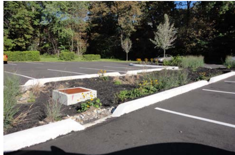
Curb cuts allow stormwater to flow into the central planting area in this parking lot in Cleveland Heights City Architecture
