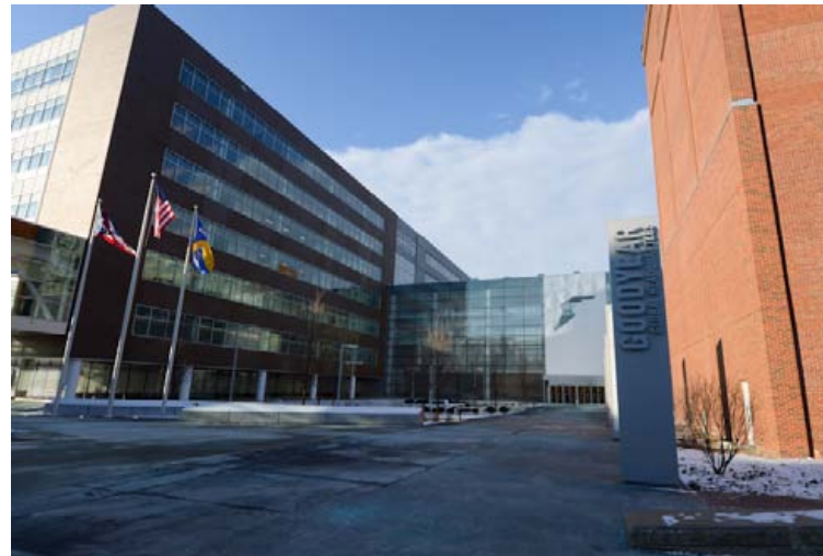
Goodyear Headquarters, Akron City Architecture
