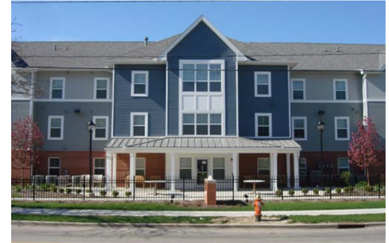
Foster Pointe, Cleveland City Architecture
