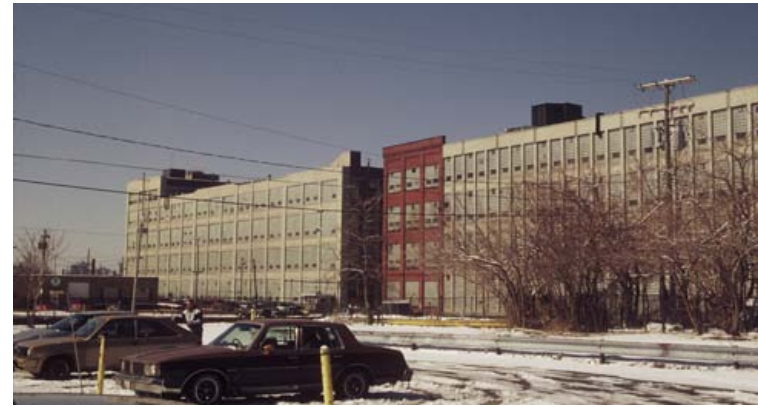
Existing Eveready Facilities City Architecture
