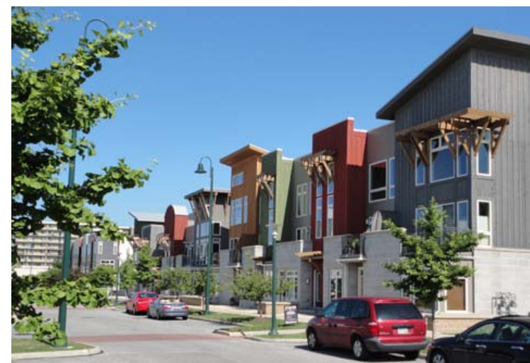
Battery Park Townhomes City Architecture
