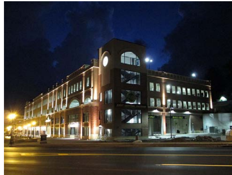
Kent Central Gateway, which opened in 2013 includes retail, bus bays, and a parking garage Photo by JonRidinger, ( http://commons.wikimedia.org/wiki/File:Kent_Central_Gateway_night_1.JPG )
