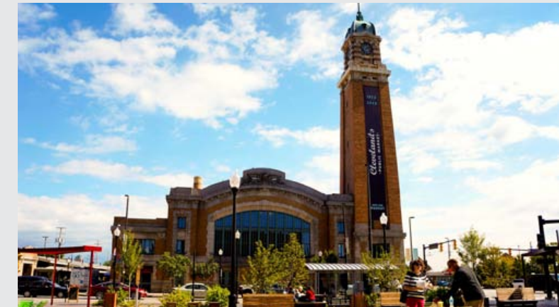
West Side Market and Market Square Park City Architecture
