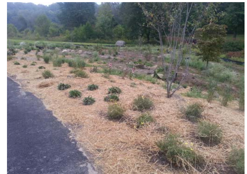
New Biofiltration Parking Lot Mill Creek MetroParks
