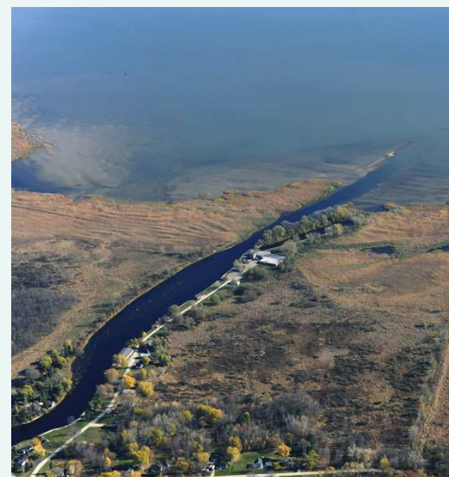
Material dredged from the Pensaukee Harbor were used to create a 4.6 acre island. Wave action has altered the original configuration into a fish-hook shape, providing habitat for birds and state-listed endangered species. It also protects from erosion by shielding an extensive wetland in the Pensaukee State Wildlife Area. (USACE)
