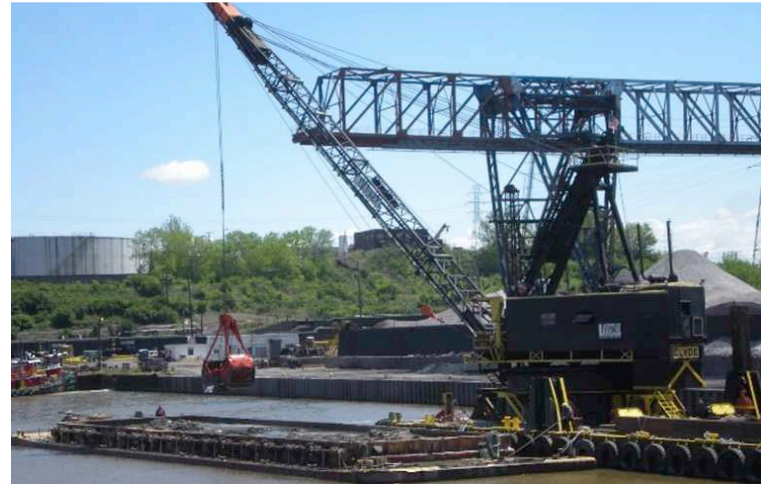
FIGURE 20. A CRANE WITH A CLAMSHELL DREDGE PLACING MATERIAL IN A DREDGE SCOW.
