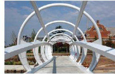
NEW PEDESTRIAN BRIDGE
