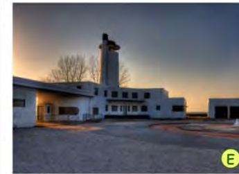
FORMER COAST GUARD STATION
