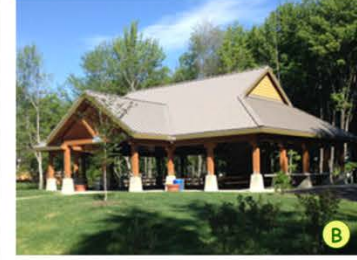
LARGE RESERVE SHELTER
