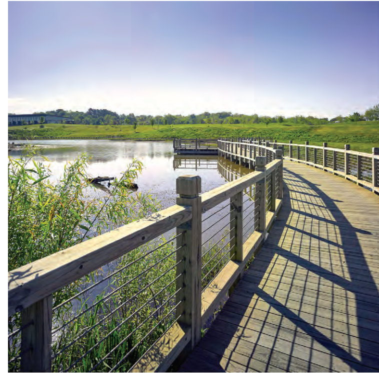
TREATMENT WETLAND WITH BOARDWALK ACCESS
