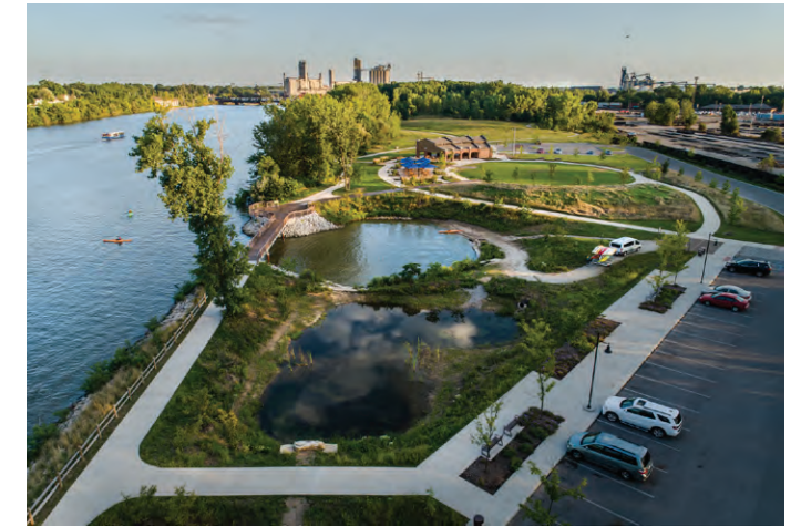
TREATMENT TRAIN CLEANING RUNOFF
