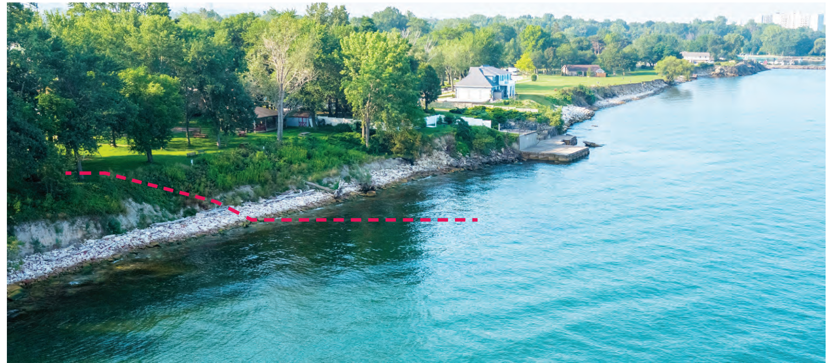
THE EASTERN PORTION OF THE COUNTY IS GENERALLY CHARACTERIZED BY SLOPING 30 - 35' BLUFFS.
